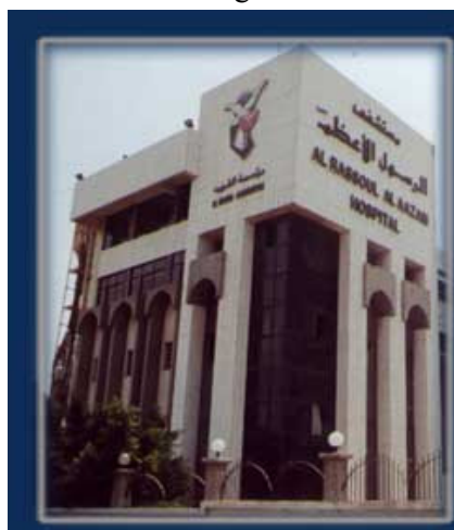
Hôpital al-Rasul al-Azam, Beyrouth-sud Source: http://www.maccorpme.com/
